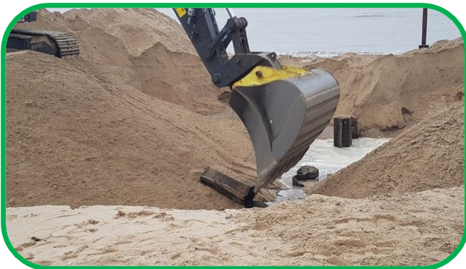
Removal of the old groynes.
